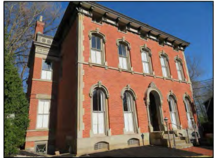
Figure 171. Site 47 (KECR 3): North and façade (west) elevations of the Hearne House, looking east-southeast.
