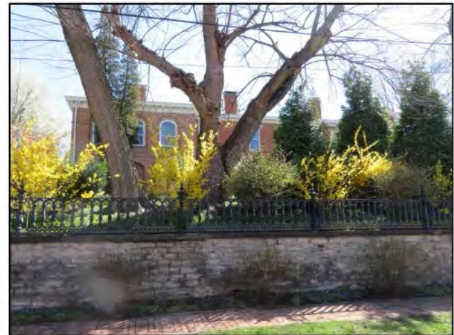
Figure 45. Site 3 (KECO 17): East elevation of the dwelling, looking west.
