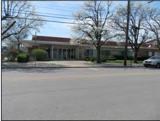
Figure 292. Site 75 (CPN 2289): View of vestibule projection, looking west.
