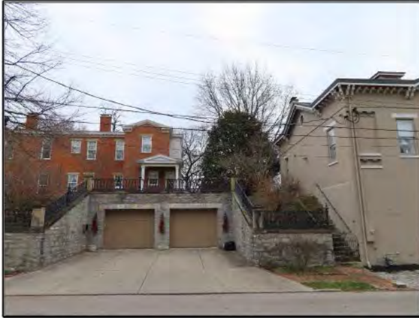
Figure 29. Site 3 (KECO 17): Image demonstrating the height of the Carneal House compared to a neighboring building.
