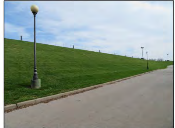
Figure 262. Site 70 (CPN 2285): Overview of levee from Riverboat Row, looking south-southeast.
