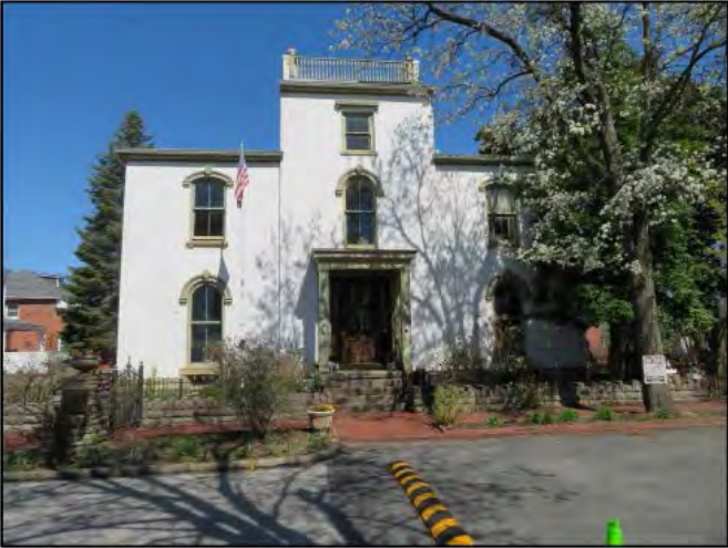
Figure 57. Site 6 (KECO 18): Façade of the dwelling, looking north.
